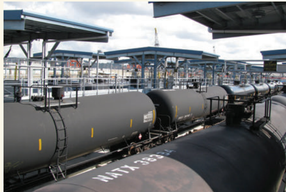
Rail loading facility.
