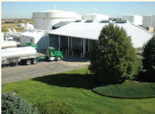
Truck loading facility.
