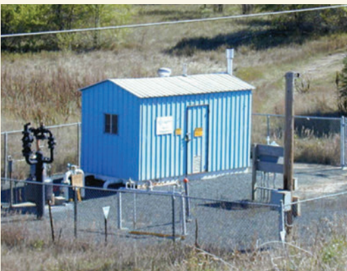
City gate meter station.
